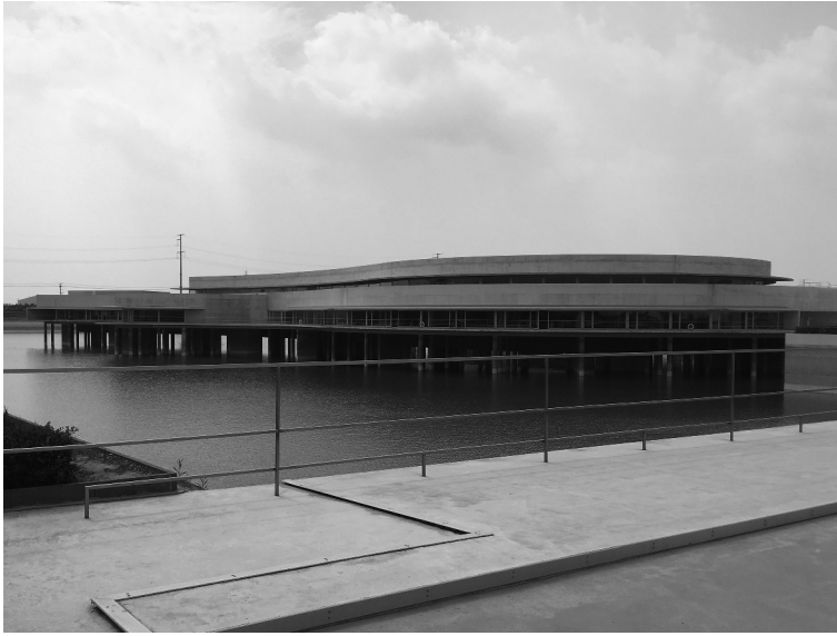
Figure 2. The first view of the Shihlien building. Photo by the author (2019).
